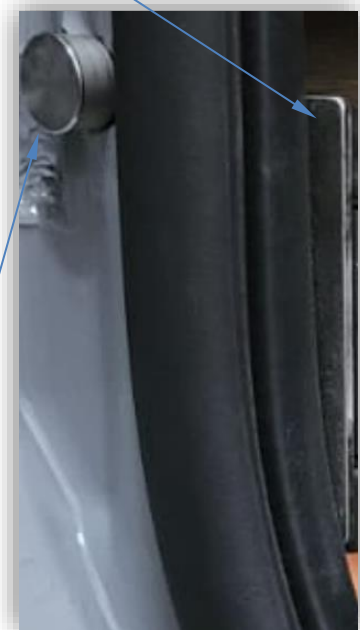
view from the outside
